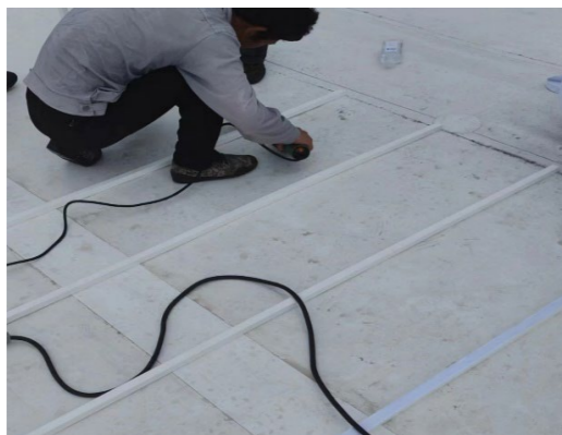
TPO 方管焊接
