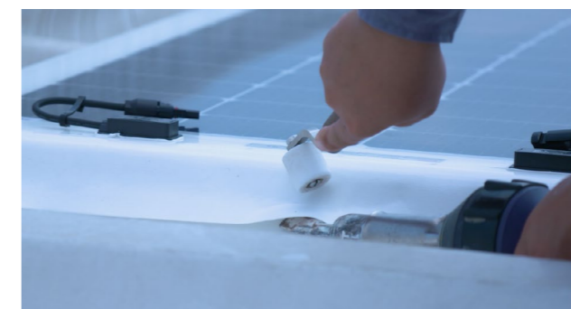
银河光伏组件热风焊接施工
